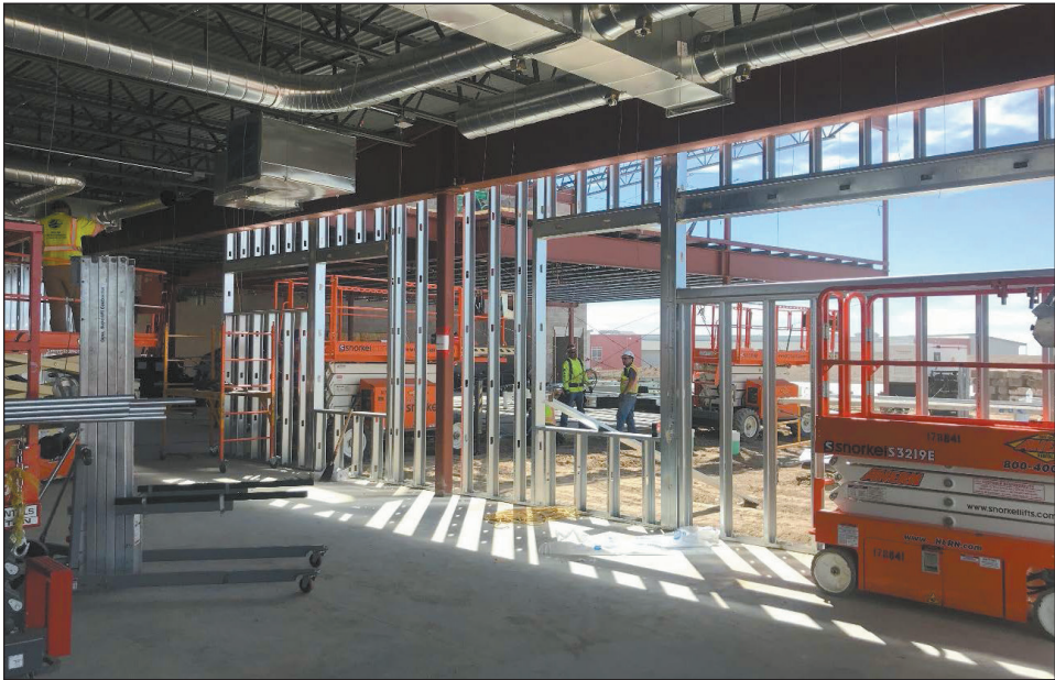
Interior framing work underway on the new D49 school on Vista Del Pico Boulevard. (Wember Inc.)
